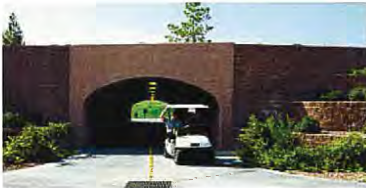
Figure 2-46A Hydro-Arch Cart Tunnel
